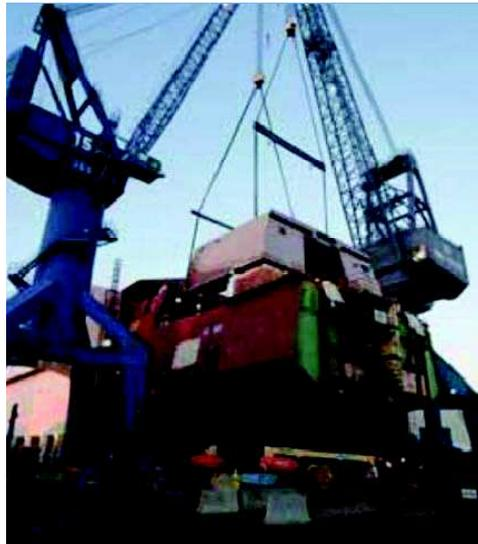
Figure 11. DDG 1000 Composite Mission Bay being integrated to the hull (Bartlett & Jones, 2013).
